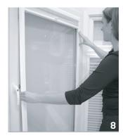
8. Fit any intermediate brackets accordingly. Clean excess lubricant from window surface prior to fixing frame to brackets.
