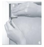
6. Line up the window fixing bracket at the base of the card (or top of the card depending upon which corner of the window you are working) and fit the bracket by pushing it between the glass and the rubber seal on the window.
